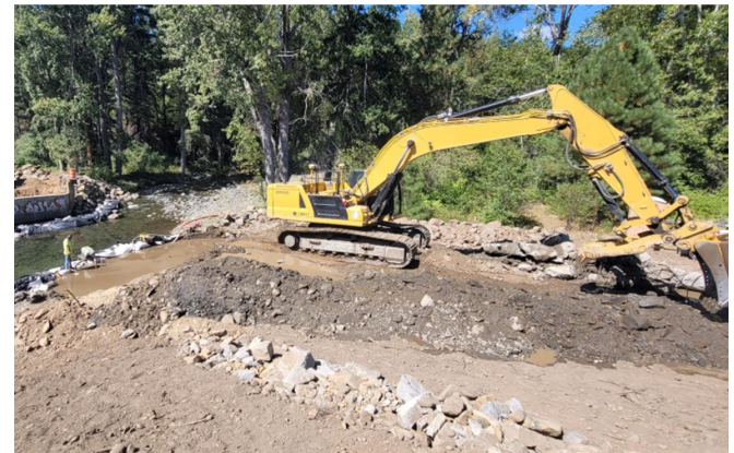
Old bridge removal
