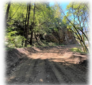
Trail being cut to sub grade
