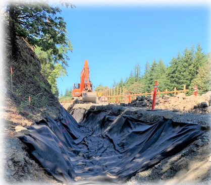
Lining ditch with geotextile separation fabric
