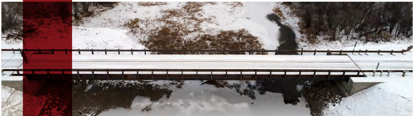
Fort Yukon Ivar’s Bridge Replacement completed. Fort Yukon, Alaska.
