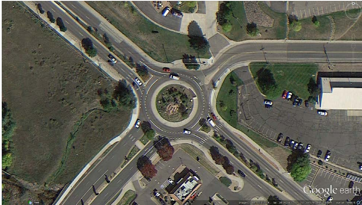
Figure 26. Photo. S. Golden Rd./Johnson St./16 th Ave., Golden, CO (Source: Google Earth 2014)
