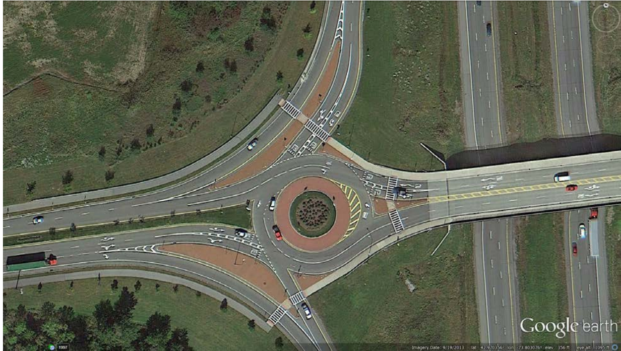
Figure 30. Photo. SR 67/I-87 SB Ramps, Malta, NY (Source: Google Earth 2013)
