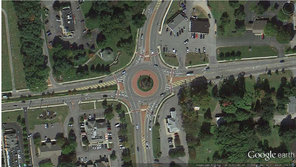
Figure 32. Photo. SR 67/US 9, Malta, NY (Source: Google Earth 2013)
