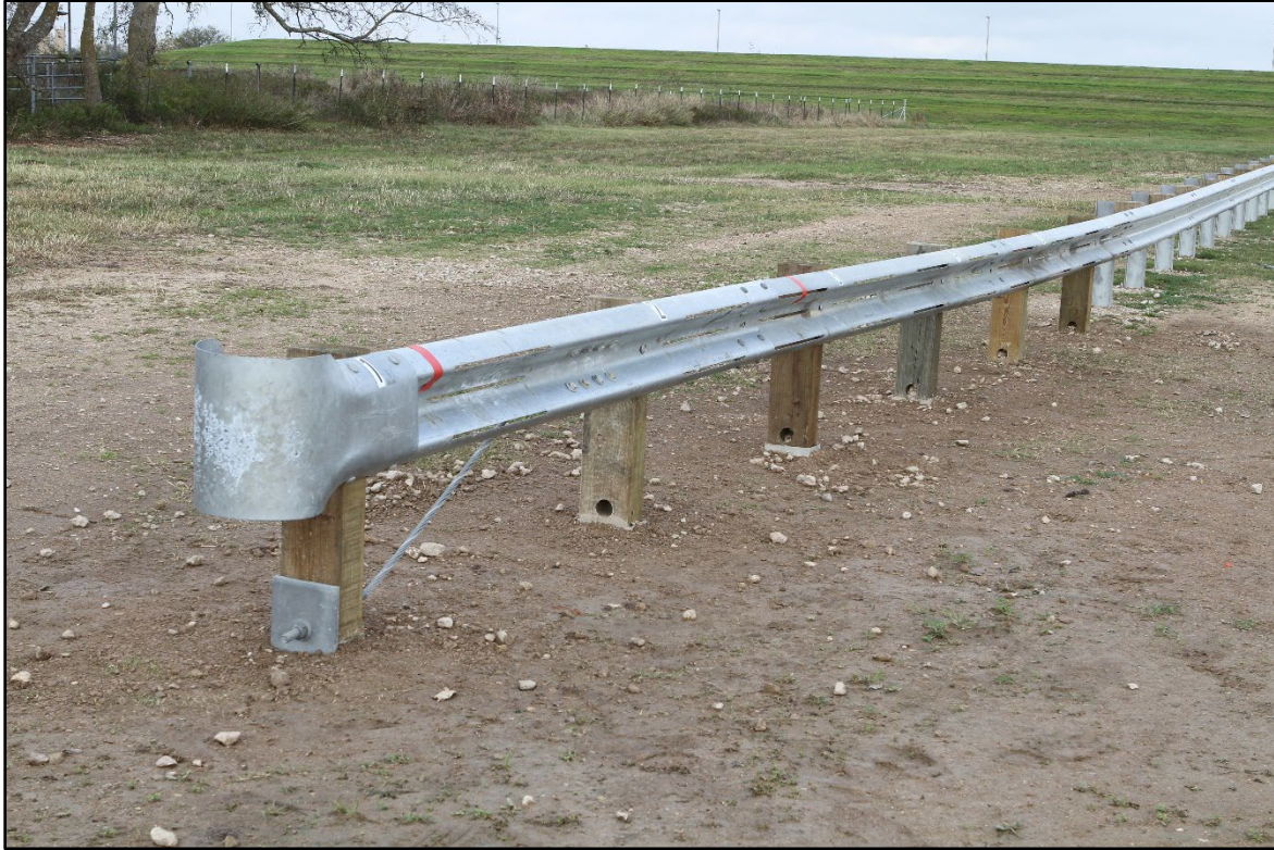
Figure 3.15. TL-2 Terminal on MGS prior to Crash Test 615181-01-10.
