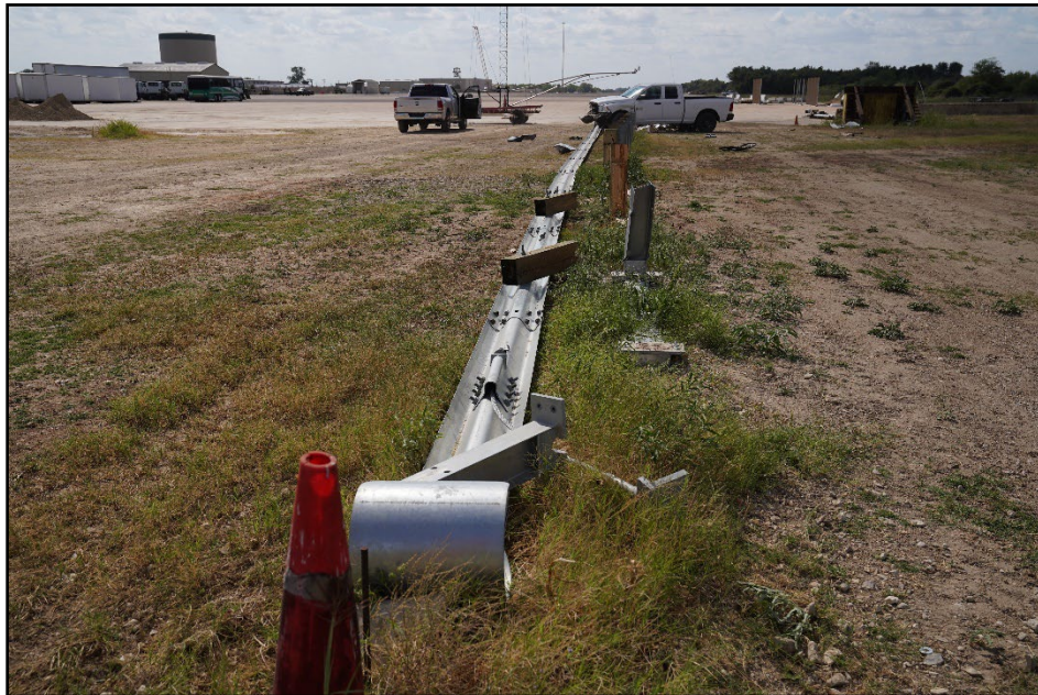
Figure 11.6. TL-2 W-beam End Terminal after Test at the Downstream Terminal 615181-01-12.
