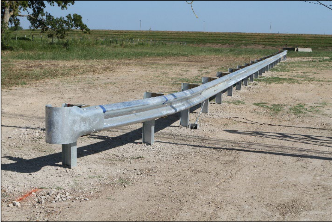
Figure 3.3. TL-2 Terminal on MGS prior to Crash Test 615181-01-1.
