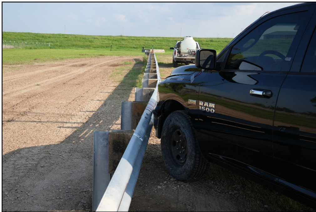
Figure 8.2. TL-2 W-beam End Terminal/Test Vehicle Impact Location 615181-01-5.
