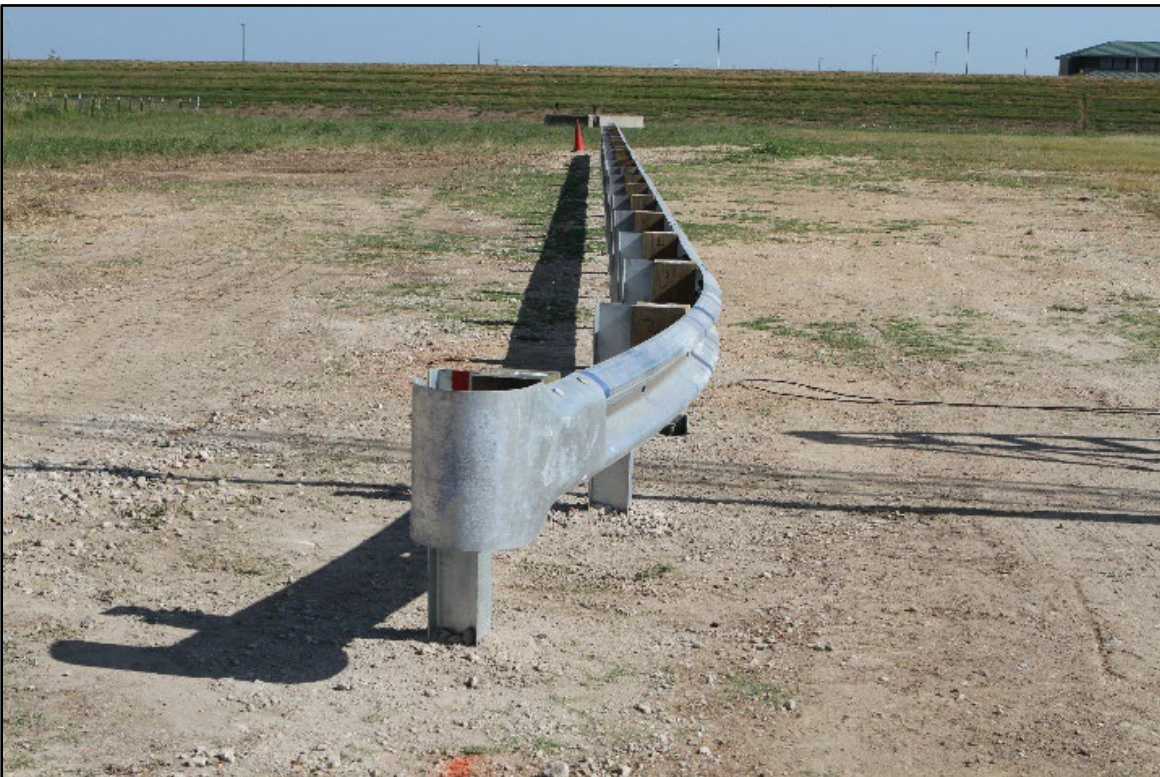
Figure 3.4. In-Line View of the TL-2 Terminal on MGS prior to Crash Test 615181-01-1.
