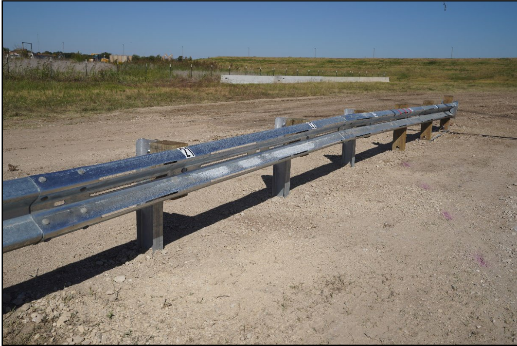
Figure 5.14. TL-2 W-beam End Terminal Prior to Test 615181-01-13.
