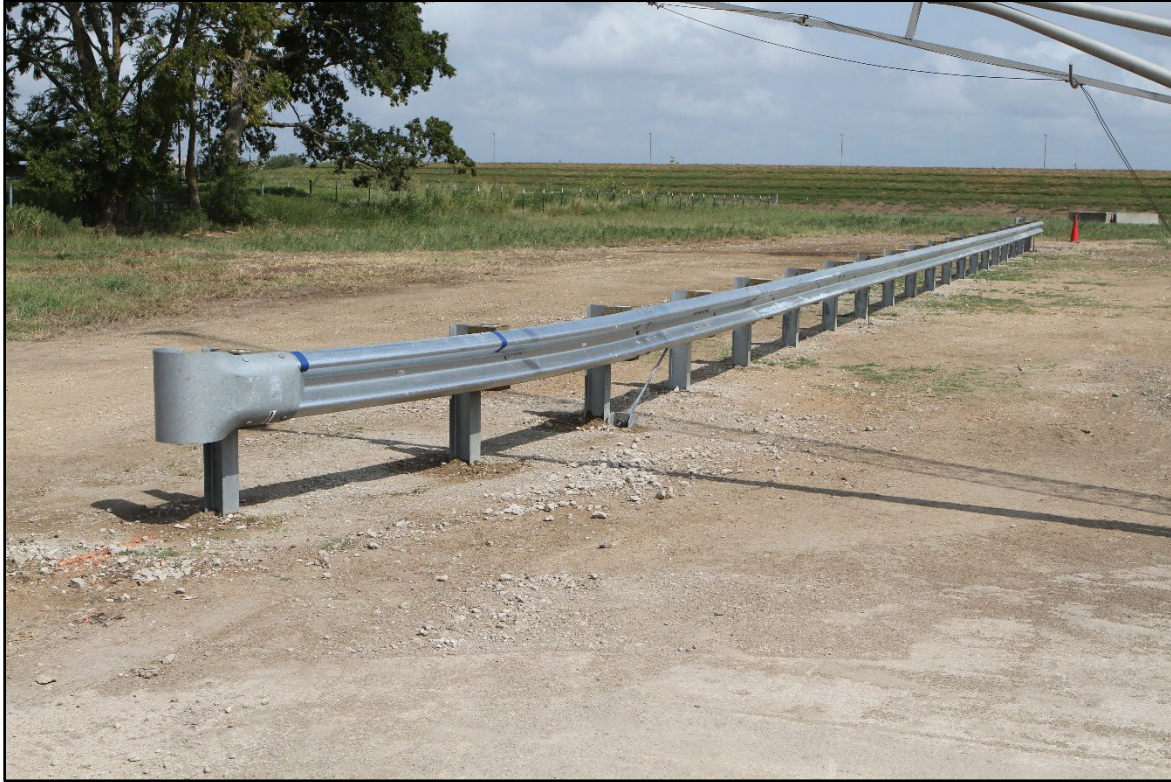
Figure 3.8. TL-2 Terminal on MGS prior to Crash Test 615181-01-2.
