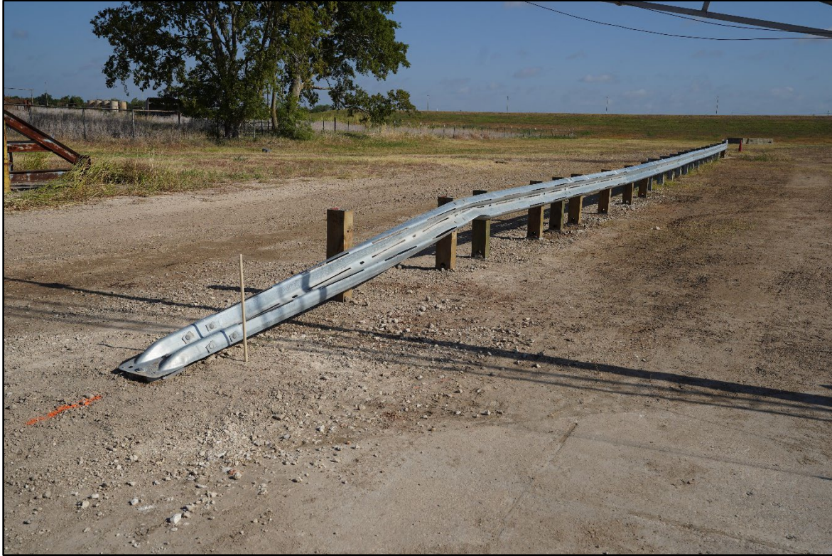
Figure 3.31. TL-2 Terminal on MGS prior to Crash Test 615181-01-3.
