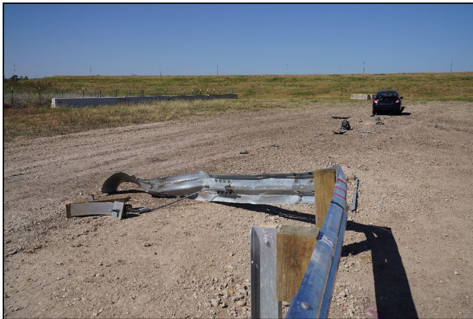
Figure 12.5. TL-2 W-beam End Terminal after Test at Impact Location 615181-01-13.
