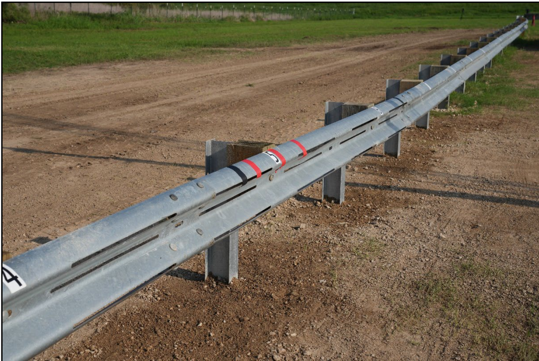
Figure 5.5. TL-2 W-beam End Terminal at Post 5 prior to Test 615181-01-5.
