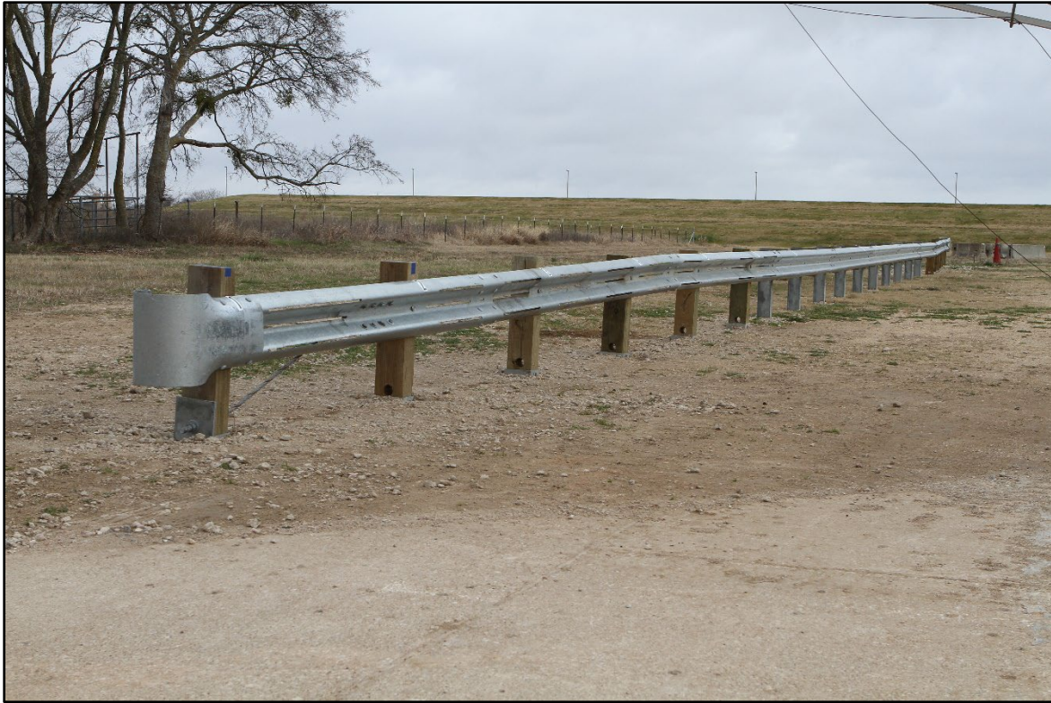
Figure 3.22. TL-2 Terminal on MGS prior to Crash Test 615181-01-9.
