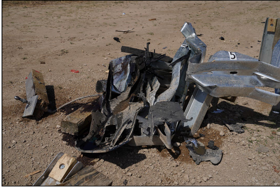
Figure 10.6. TL-2 W-beam End Terminal after Test after the Small Car was Removed 615181-01-11.
