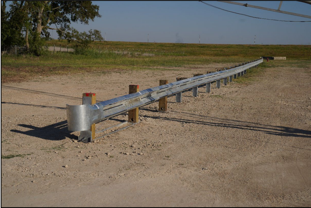
Figure 5.9. TL-2 W-beam End Terminal prior to Tests 615181-01-11 & 615181-01-12.
