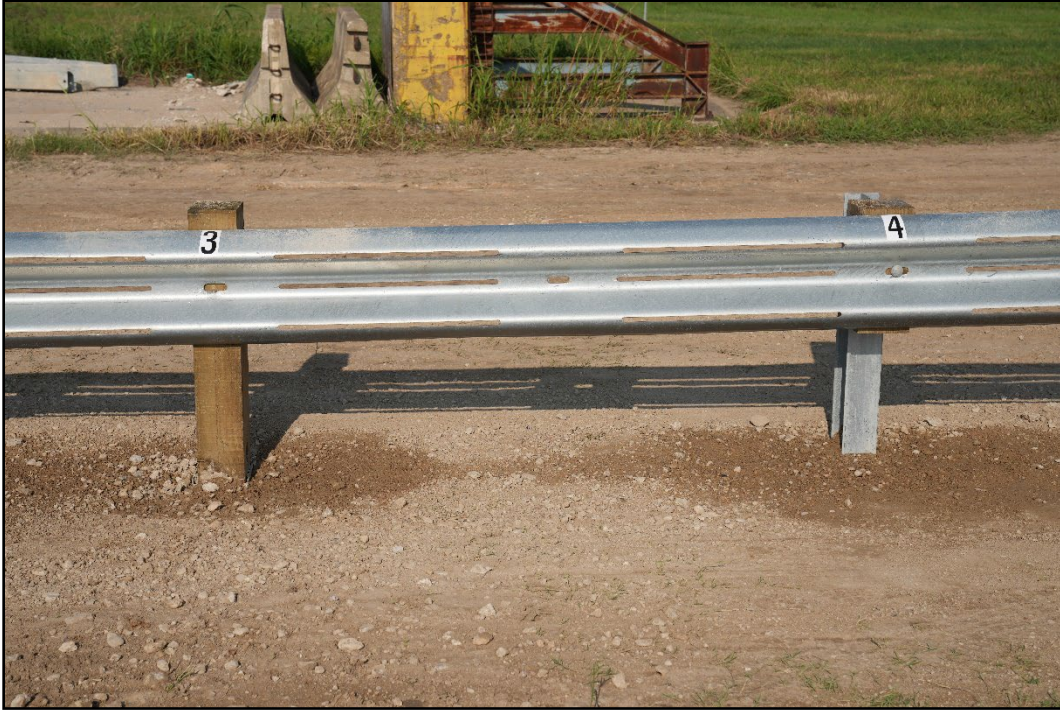
Figure 5.4. TL-2 W-beam End Terminal at Posts 3 and 4 prior to Test 615181-01-5.
