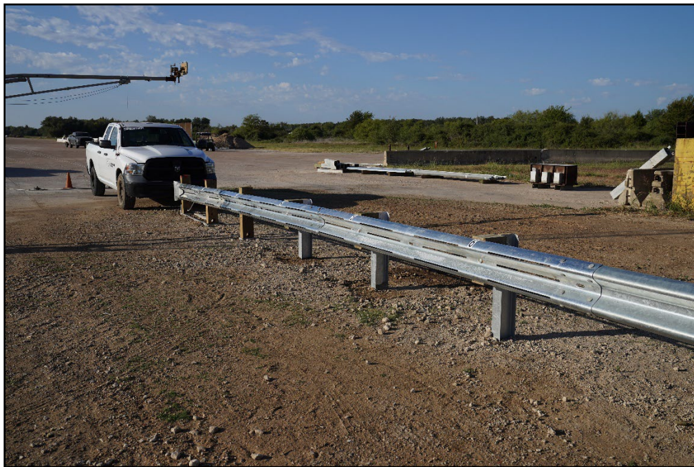
Figure 11.2. TL-2 W-beam End Terminal/Test Vehicle Impact Location 615181-01-12.
