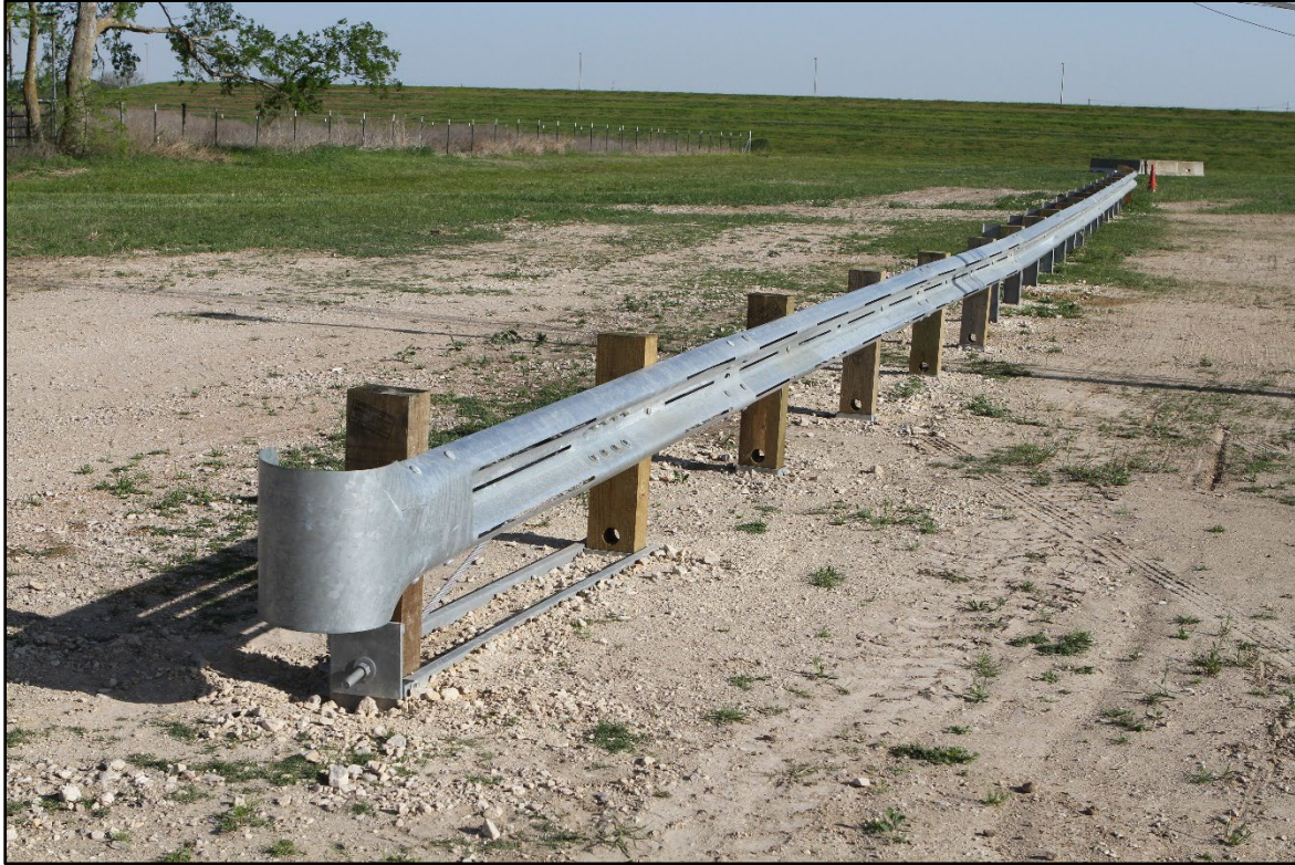
Figure 3.27. TL-2 Terminal on MGS prior to Crash Test 615181-01-8.
