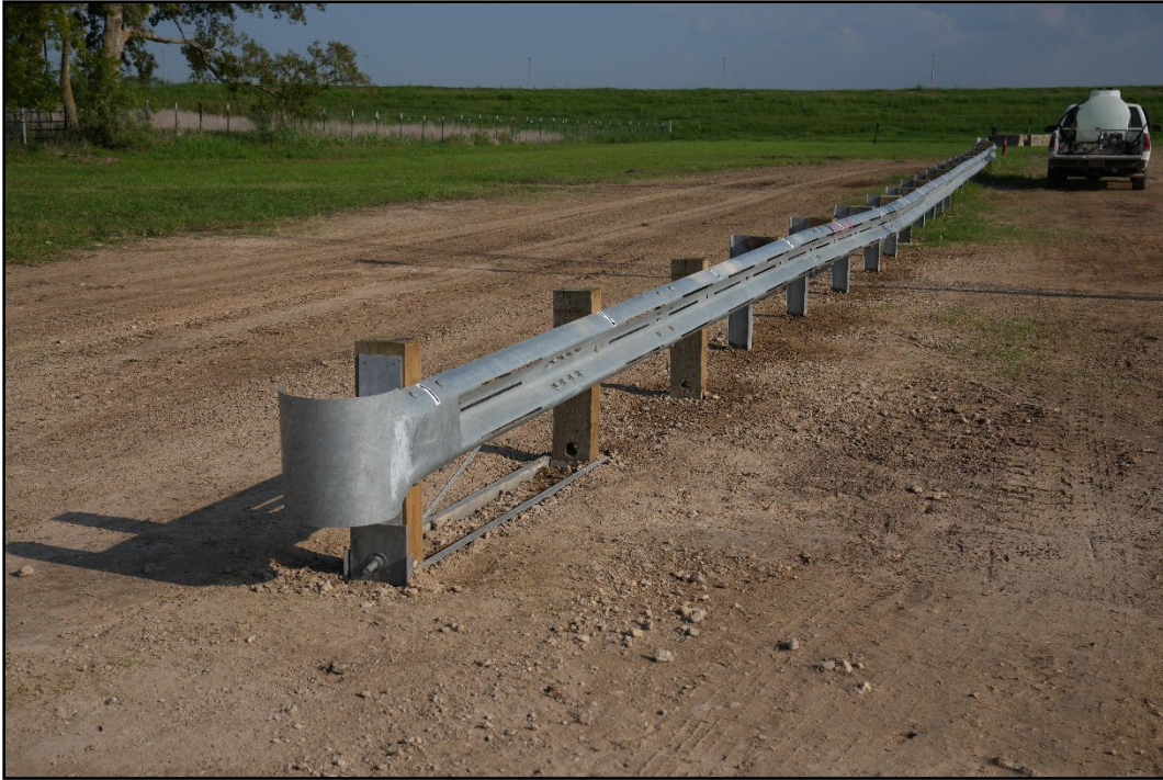
Figure 5.2. TL-2 W-beam Installation prior to Test 615181-01-5.
