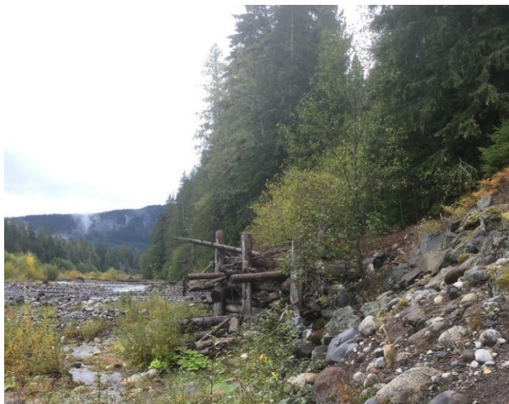
Figure 3-12: Mount Rainier National Park Roadway Erosion Reduction Measures: Engineered Log Jam
