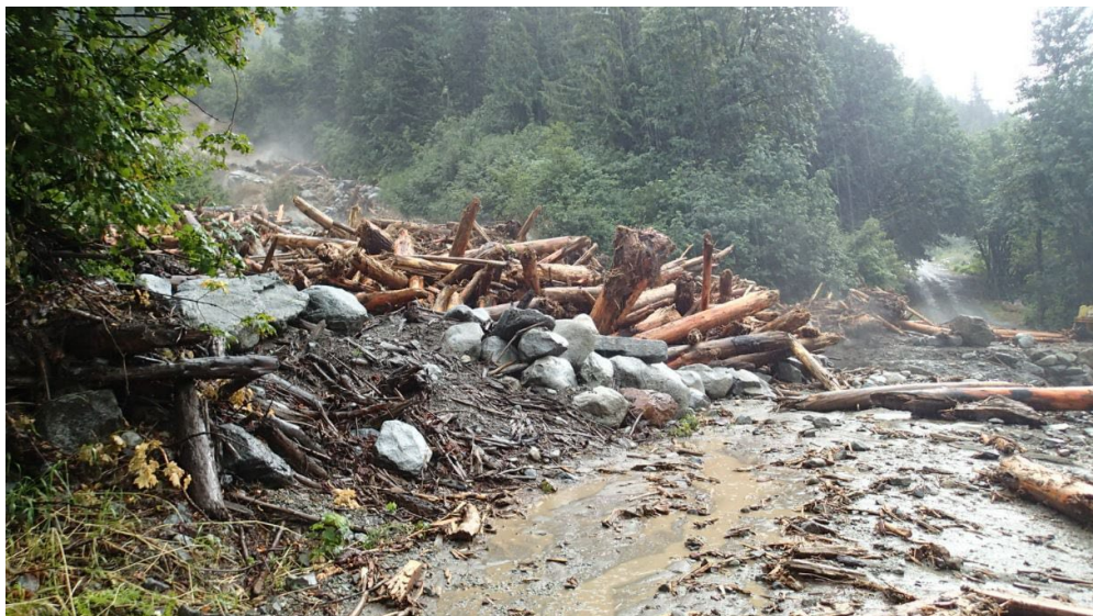
Figure 3-6: The Impact of a Flood on Cascades River Road
