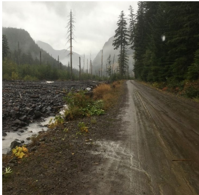
Figure 3-11: Mount Rainier National Park Road with Engineered Log Jam Foundation
