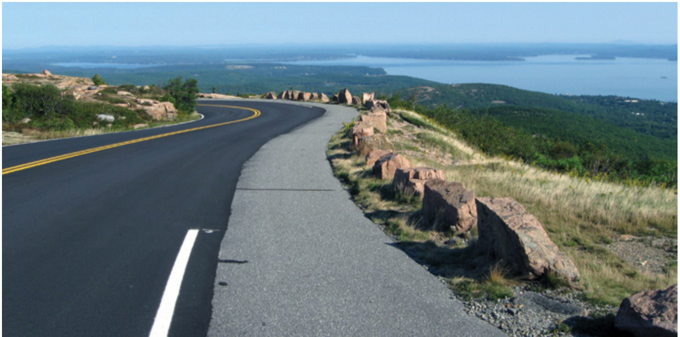
Cadillac Mountain Road, Acadia National Park. Photo by VHB.
