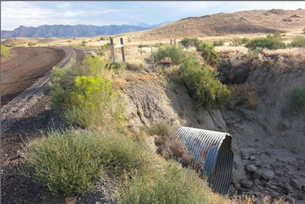
Figure 11. 18 Mile Road before construction of improvements in Colorado
