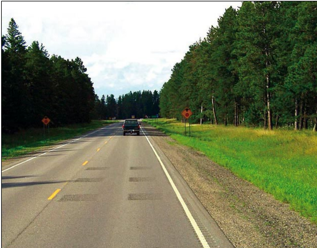
Figure 85. Photograph. Example of transverse rumble strips on a rural road. (69)
