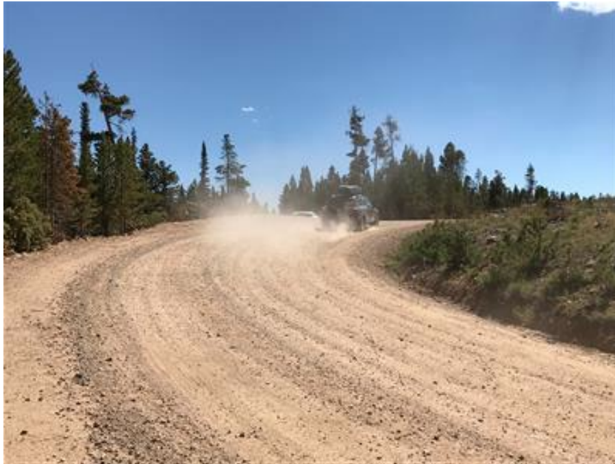
Figure 94. Photograph. Vehicle turning and demonstrating the horizontal curve and visual trap in figure 93.
