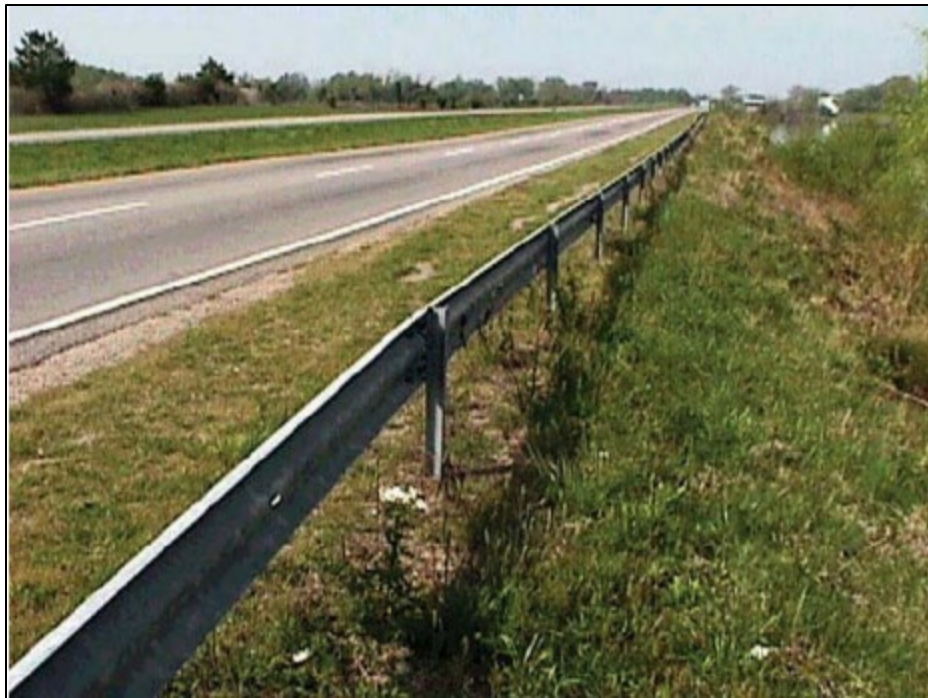
Figure 75. Photograph. Example weak post w-beam. (59)
