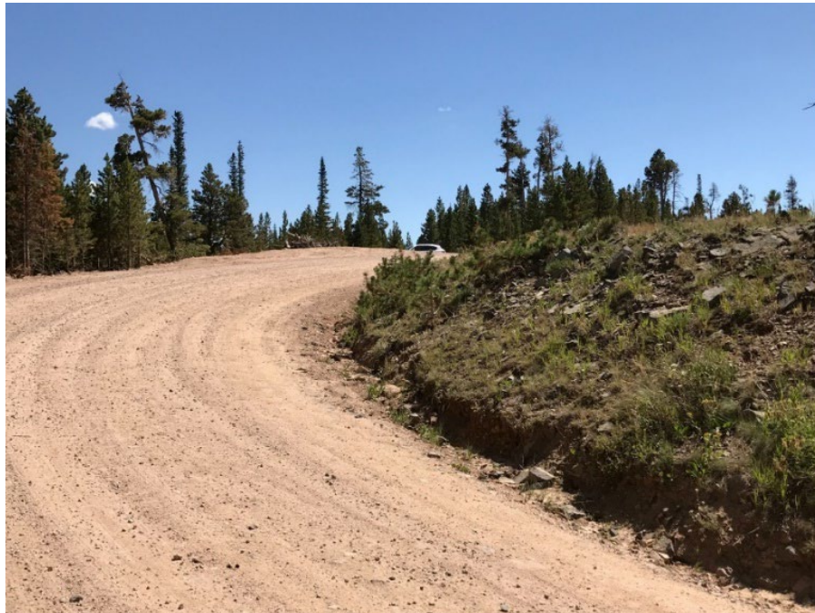
Figure 93. Photograph. Break in the tree line providing a visual cue that can be a potential visual trap.
