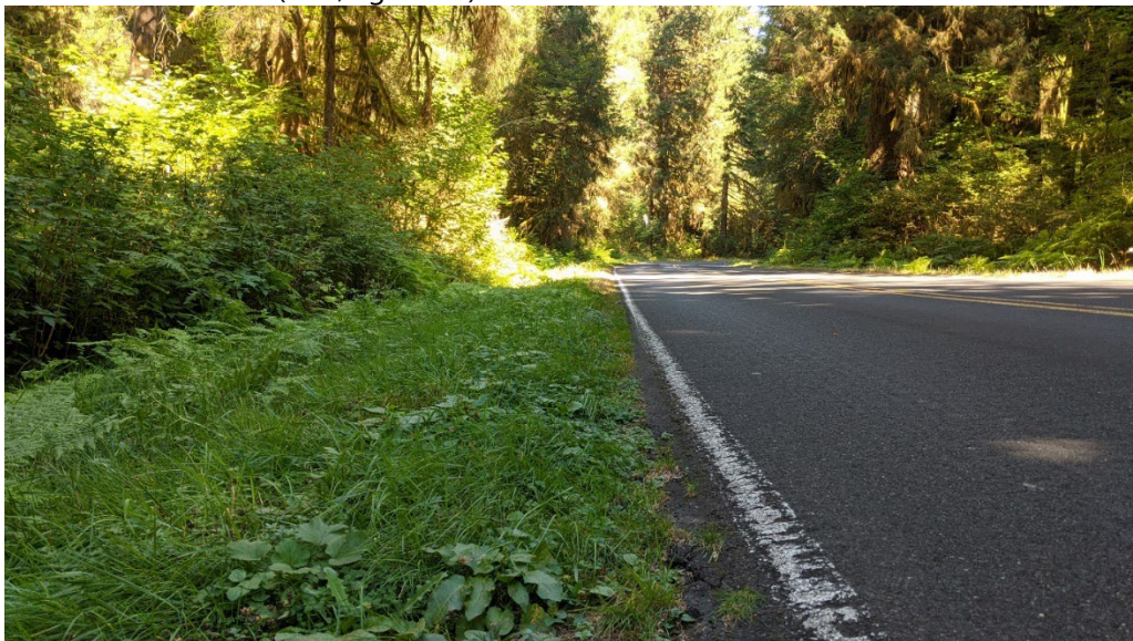
Figure 28. Photograph. Narrow and unpaved shoulder.
