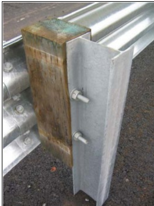
Figure 71. Photograph. Example strong post w-beam. (59)
