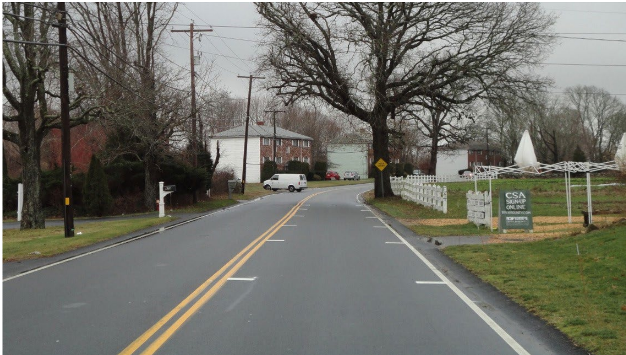
Figure 87. Photograph. Example of optical speed bars. (65)
