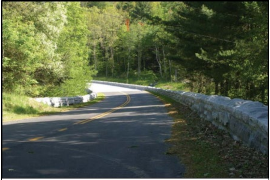
Figure 98. Photograph. Example stone masonry guardwall. (59)
