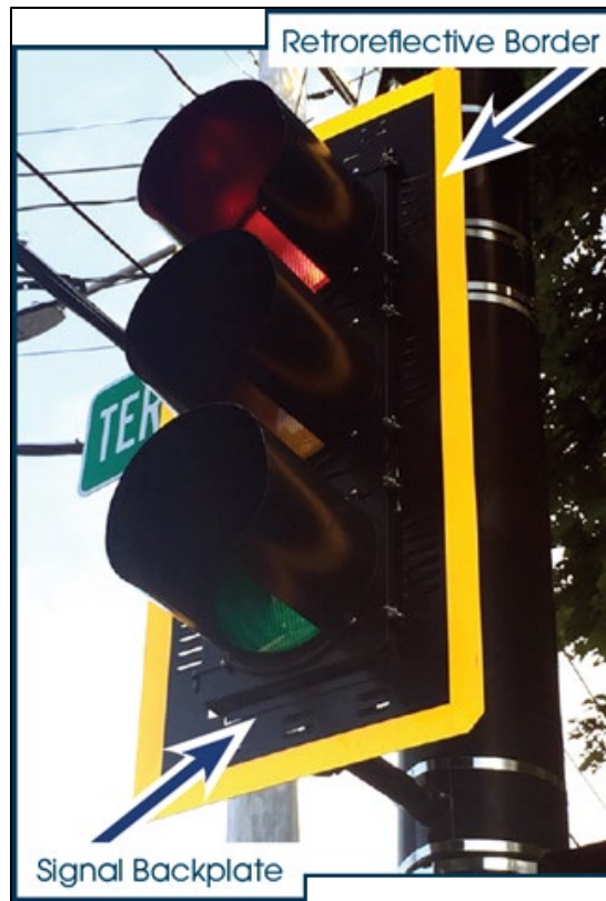
Figure 86. Photograph. Example of retroreflective back plate. (70)
