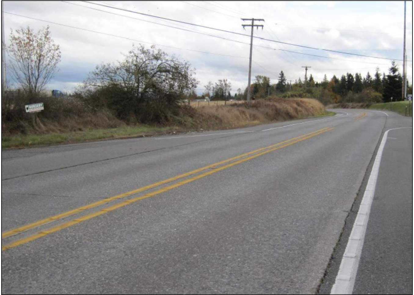
Figure 82. Photograph. Example of profile thermoplastic pavement markings. (66)
