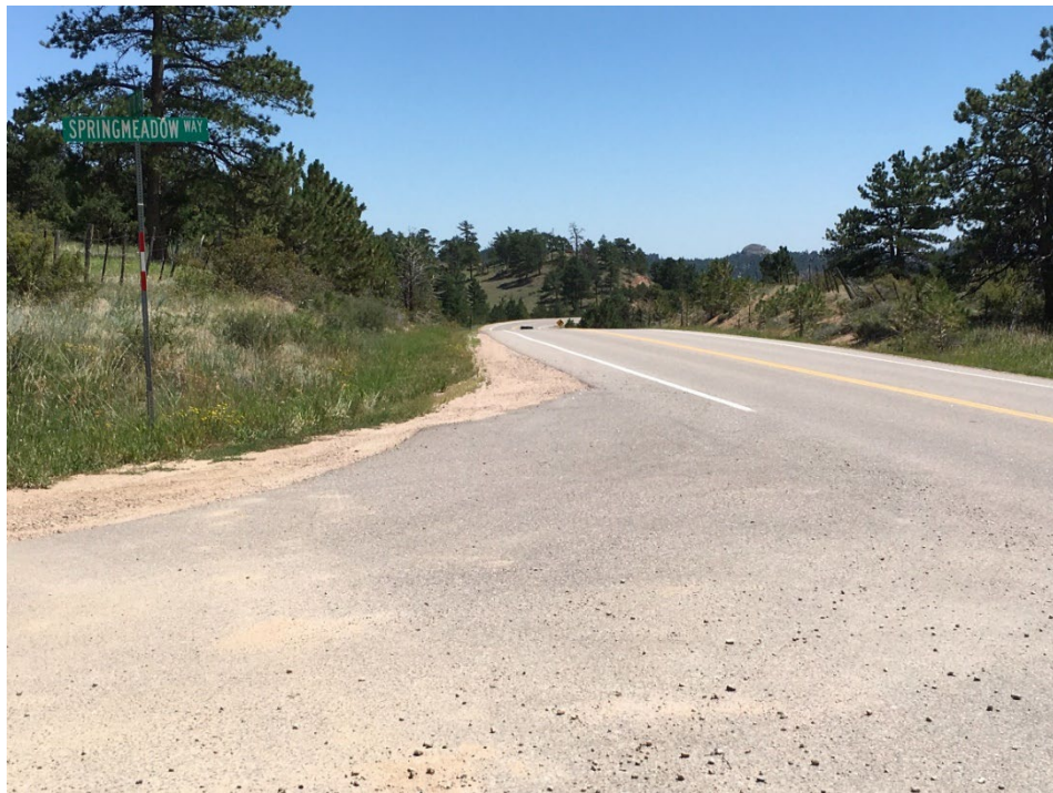
Figure 33. Photograph. Vehicle entering a vertical curve with substantial vertical grade.
