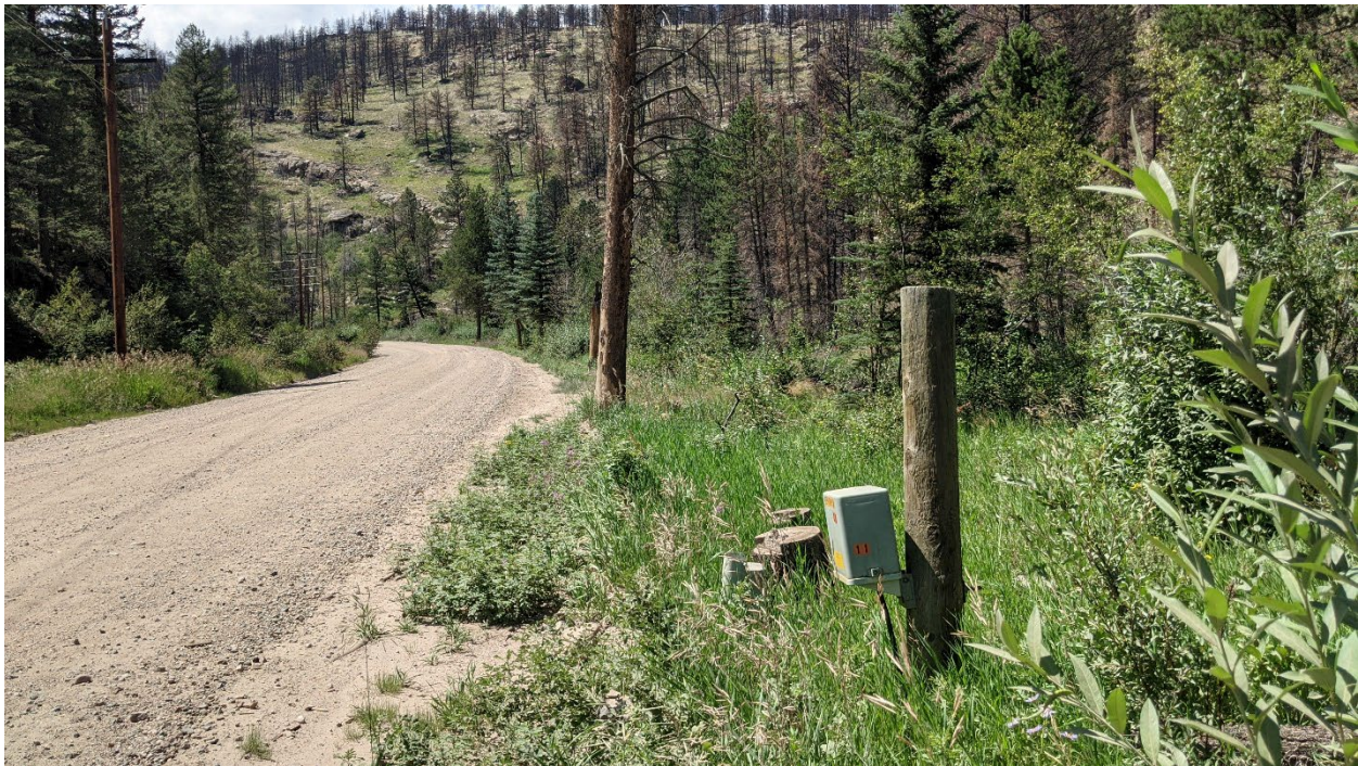
Figure 35. Photograph. Example of fixed objects less than 3 ft from the edge of the road.
