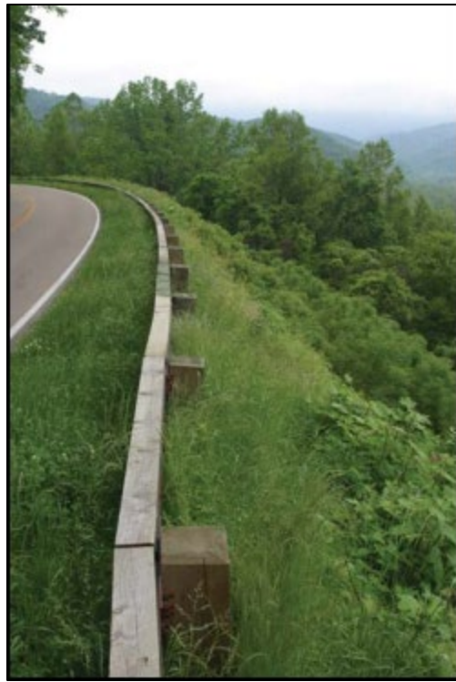
Figure 69. Photograph. Example steel-backed timber rail. (59)
