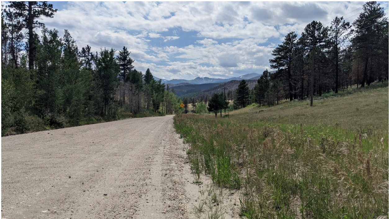
Figure 36. Photograph. Example of fixed objects 3 to 15 ft from the edge of the road.
