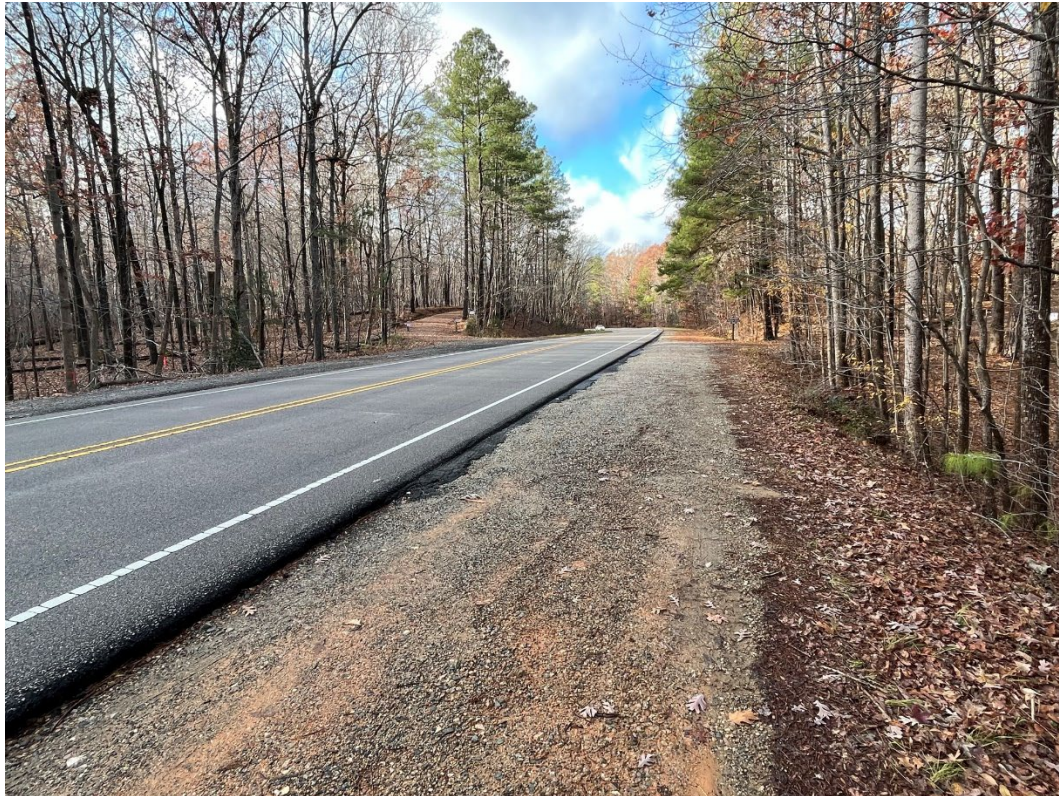
Figure 57. Photograph. Example of a pavement drop off.
