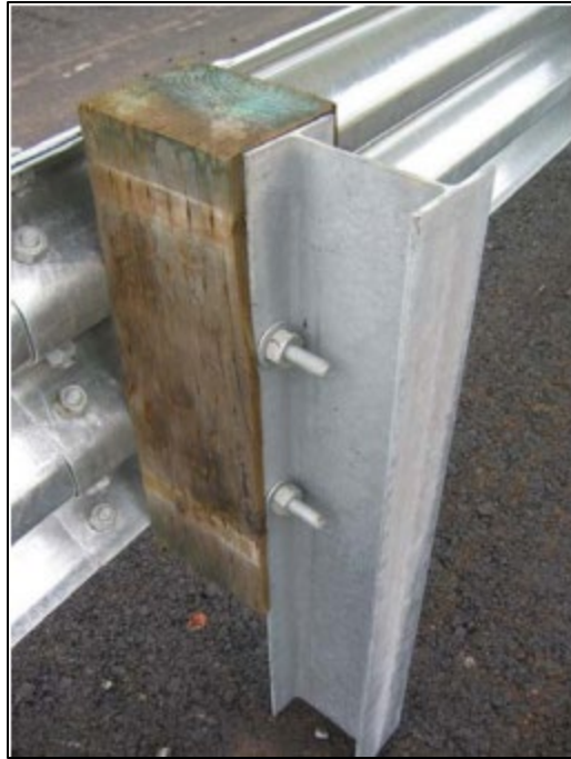
Figure 102. Photograph. Example thrie-beam. (59)
