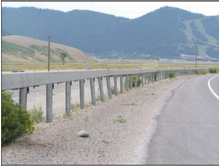
Figure 100. Photograph. Example box beam. (59)
