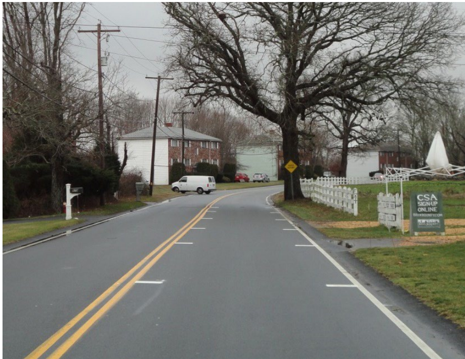
Figure 63. Photograph. Example of optical speed bars. (65)
