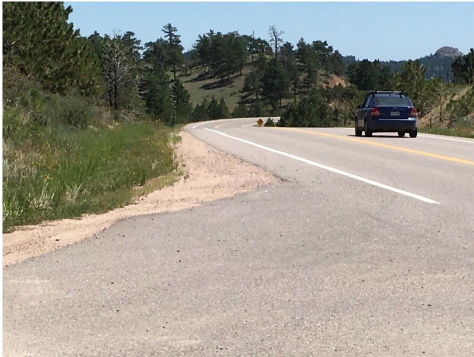
Figure 33. Photograph. Vehicle entering a vertical curve with substantial vertical grade.
