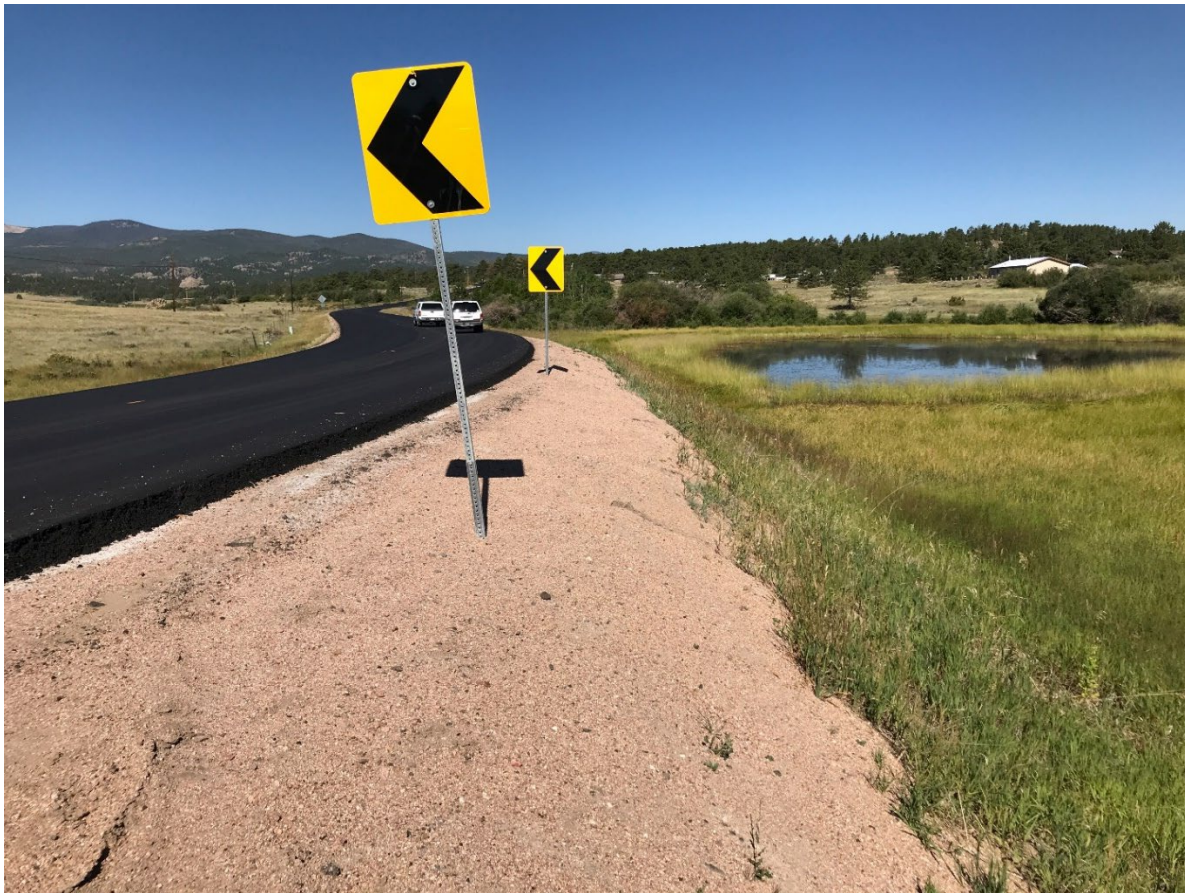
Figure 31. Photograph. Example of curve chevrons providing adequate delineation on a horizontal curve.
