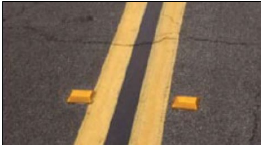
Figure 88. Photograph. Example of raised pavement markers. (67)
