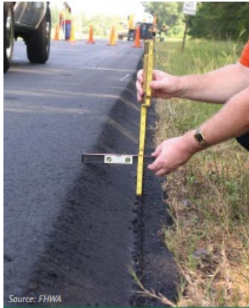
Figure 109. Photograph. SafetyEdge SM example. (68)
