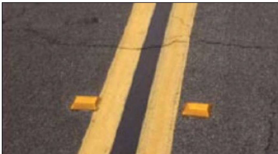
Figure 64. Photograph. Example of profile thermoplastic pavement markings. (66)
