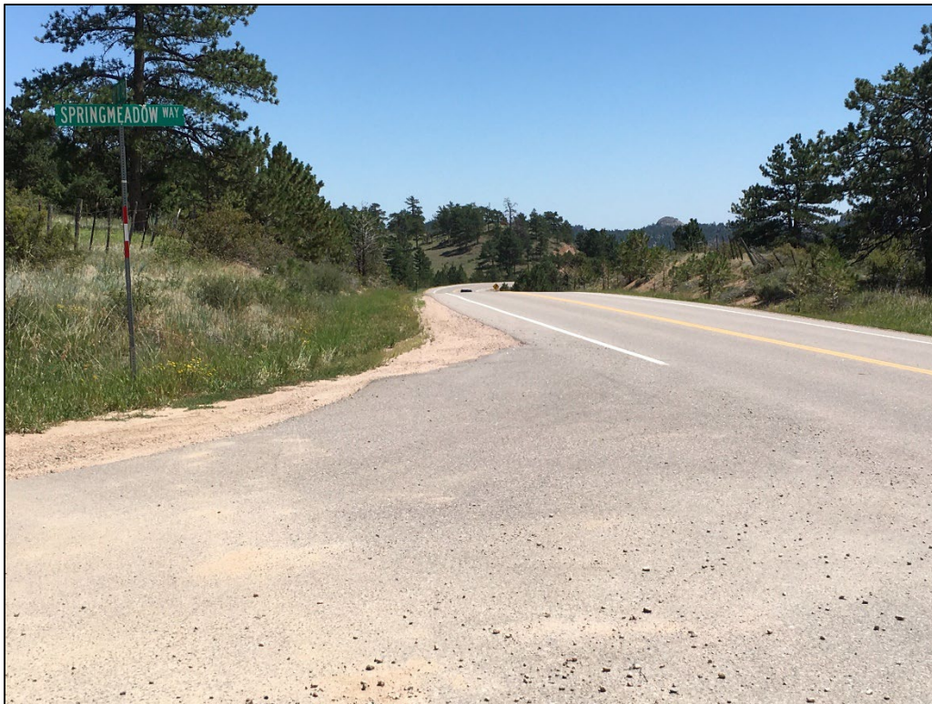
Figure 91. Photograph. Vehicle obscured by vertical curvature at the same location in figure 90.
