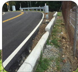
Geosynthetic-Reinforced Soil with Concrete Masonry Units used to build embankment
