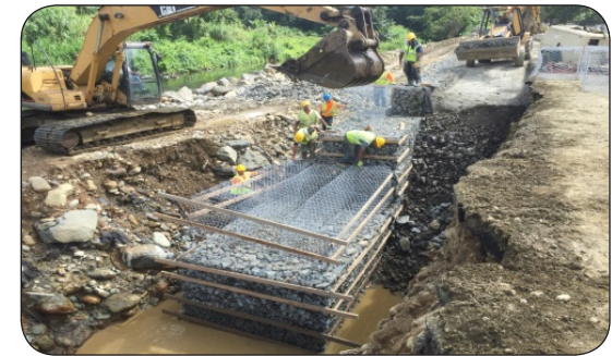
Gabion Wall Construction
