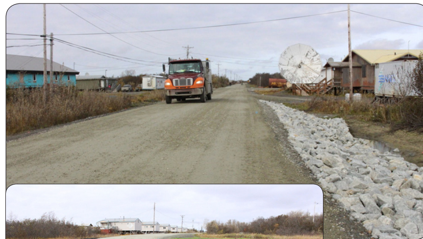
Finished roadbed showing riprap fillslope protection and (left) view of raised road and riprap culvert inlet.
