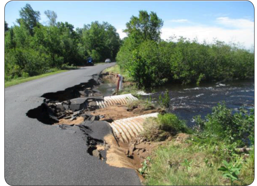
Views of road and culvert damage — Forest Service Road 194, Chequamegon-Nicolet National Forest
