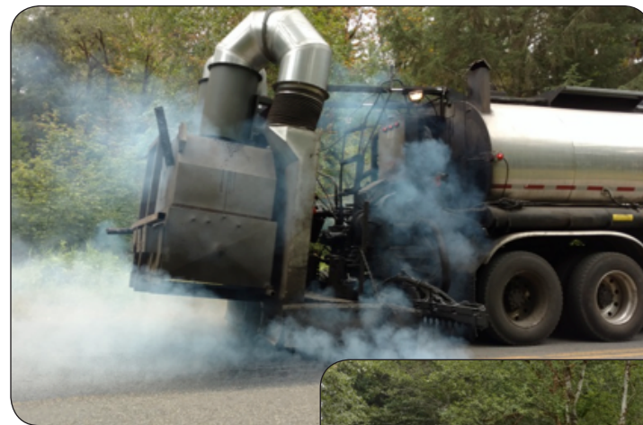
Chip Seal Application — Cispus Road, Gifford Pinchot National Forest, Washington
