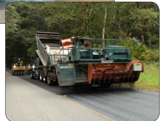
Chip Seal Application — Cispus Road, Gifford Pinchot National Forest, Washington
