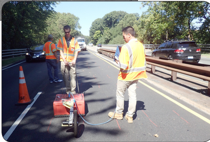
FLH Geotechnical engineers employ the use of Ground Penetrating Radar to evaluate subsurface conditions and identify areas prone to soil loss in order to minimize future sinkhole formation along the Parkway
