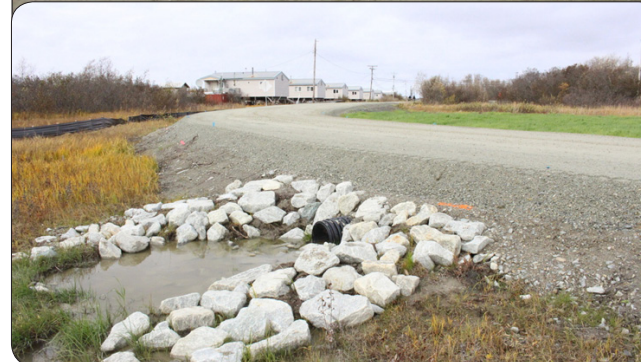
Finished roadbed showing riprap fillslope protection and (left) view of raised road and riprap culvert inlet.
