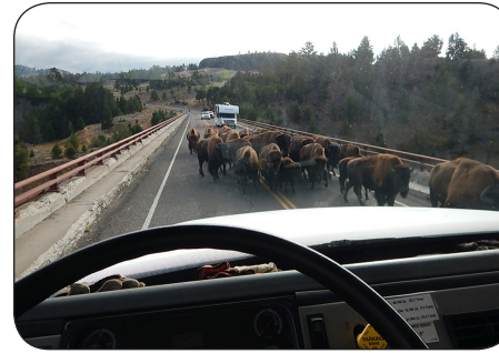
Traffic control during inspections is not always effective with the locals! — image captured from inside the "Snooper" inspection vehicle — Yellowstone River Bridge, Wyoming
