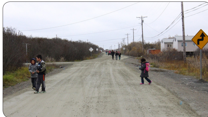
School children and other local residents make use of their newly reconstructed road.
