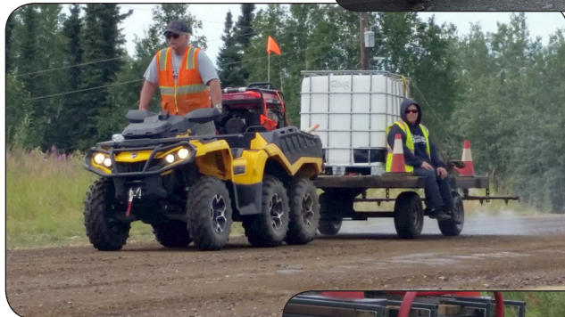
Palliatives being applied to road surface
