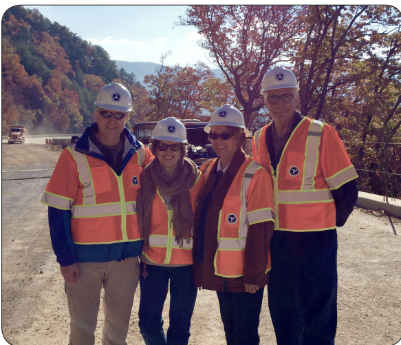
Onsite at Foothills Parkway bridge construction site, Great Smoky Mountains National Park, Tennessee (left to right) Tim Hess with Sandy Otto, Director Western Federal Lands; Melisa Ridenour, Director Eastern Federal Lands; Ric Suarez Director Central Federal Lands.
