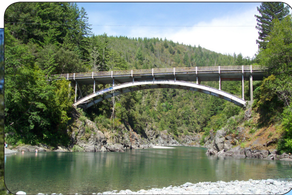
View of the original bridge.
