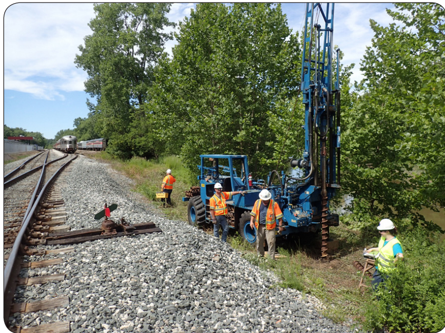
FLH Drill Crew installing slope inclinometer to monitor ground movement
