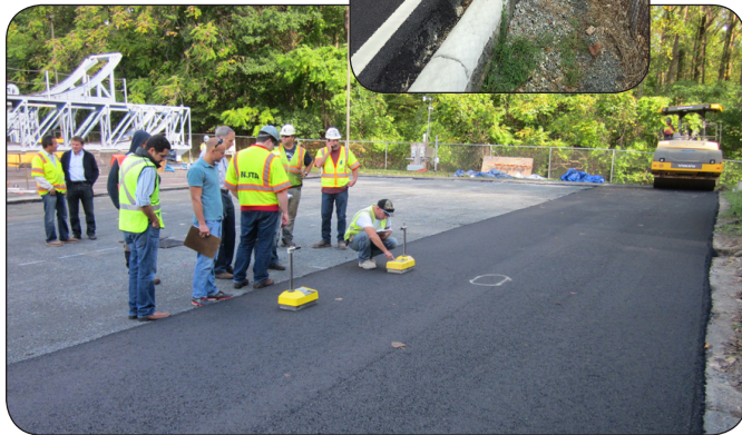
New pavement at the Asphalt Testing Facility, TFHRC, McLean, Virginia
