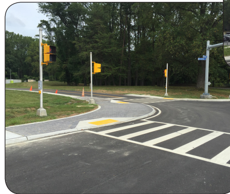
Views of the new intersection constructed with alternative construction materials
