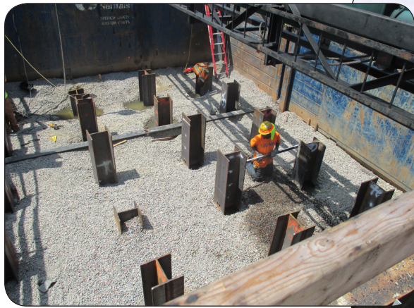
Fence posts for the Navy Security Perimeter Fence
